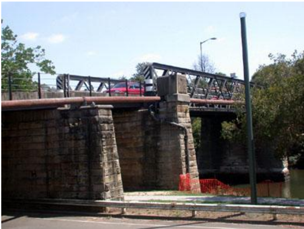
Figure 4 – Gasworks Bridge (formerly Newlands Bridge), photographed c. 2004 ( http://www.heritage.nsw.gov.au/07_subnav_01_3.cfm?itemid=2240221&imageid=2240245 )
