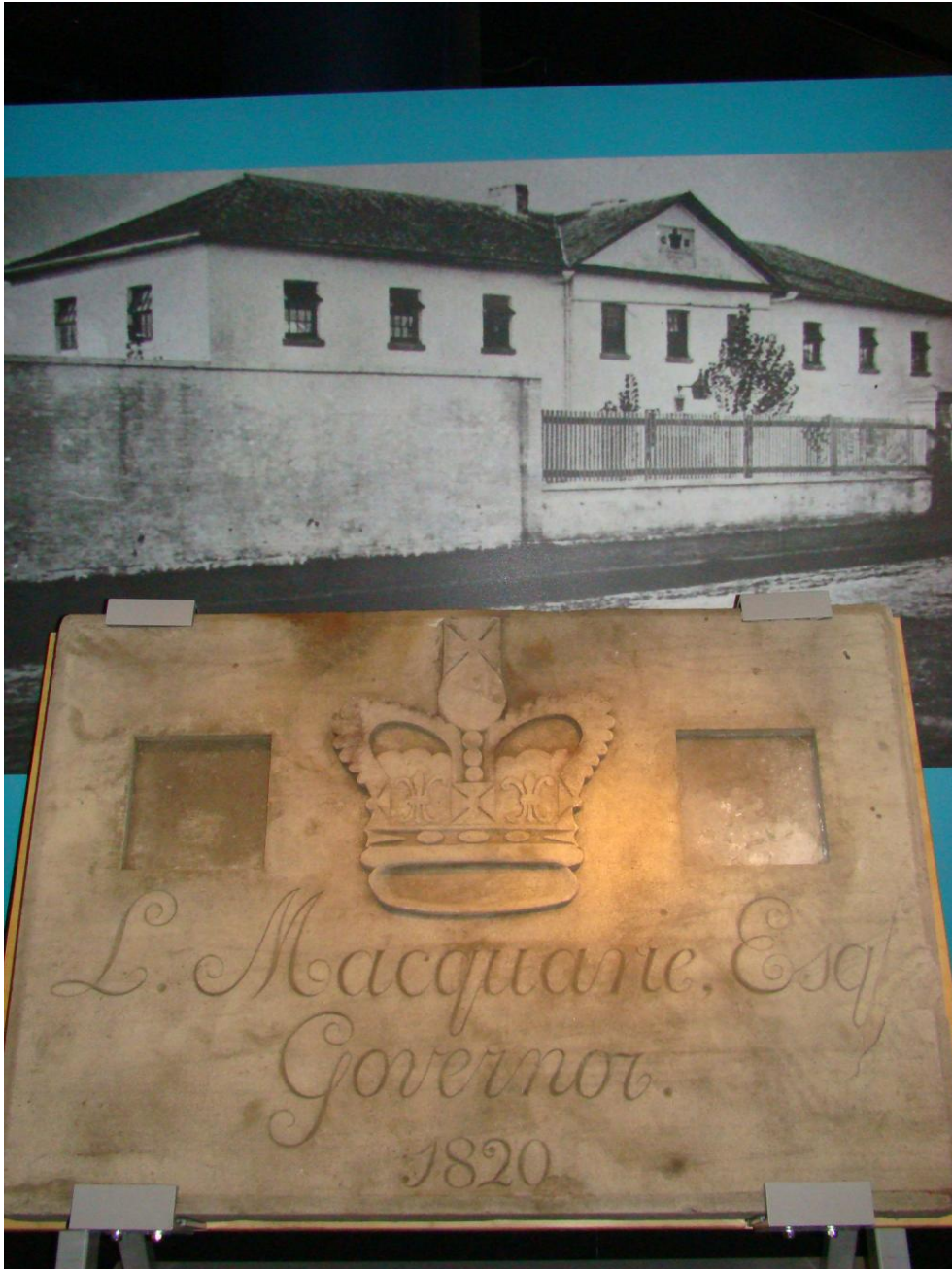
Figure 2 – “Foundation stone” (pediment stone) from Convict Barracks, photographed in Council’s Heritage Centre in Church Street, 2012. The stone is on public display with a historical context photograph interpreting its original place on the Convict Barracks building
